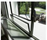
Steel hopper windows open inward from the bottom frame and are often found in settings with restricted exterior projection.
